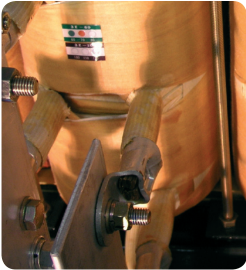
Legend Power's Electrical Harmonizer – AVR reduces energy consumption by 6-10%.
